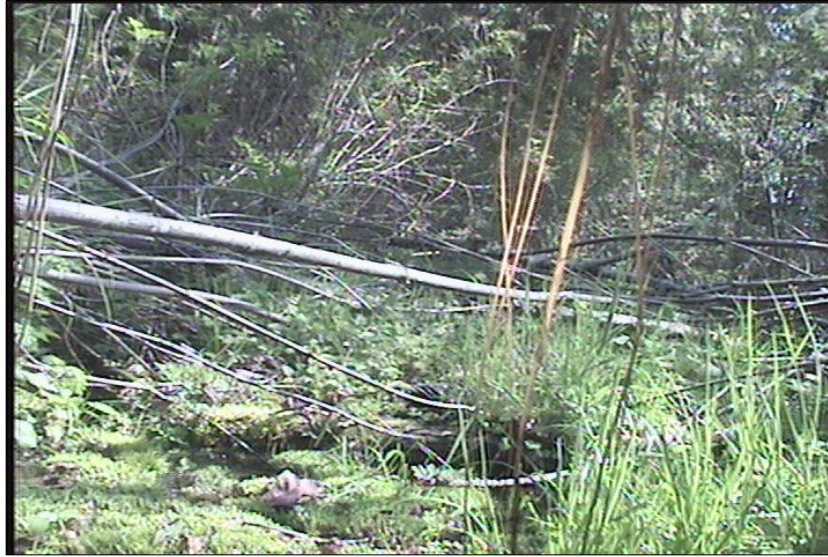
Photo: INLET-W_OUTLET103021_19052011_A.JPG, VCR No.: 1 63.12FT, End of Pipe
